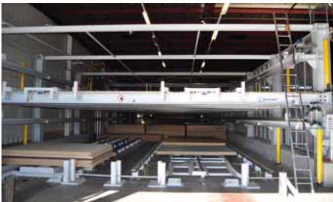
Top: Albert Nopp, production manager at Hali, with Josef Lindinger, operator of the Holzma HKL 380 CombiLine angular system.
