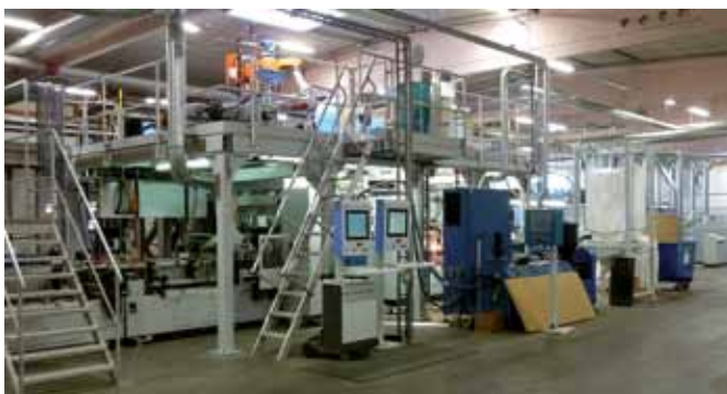
Right: Complete line, finish processing in the foreground
