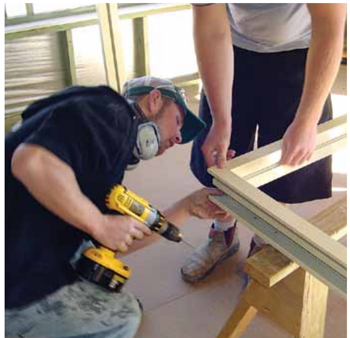
Wagga Wagga shopfitting student Ben Wealands assembles an aluminium shopfront frame.
