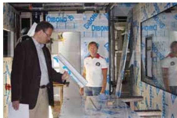
Below: Here you can see a rolling biometric lab destined for use in Africa. Internal cladding of the walls: dibond aluminum composite panels.
