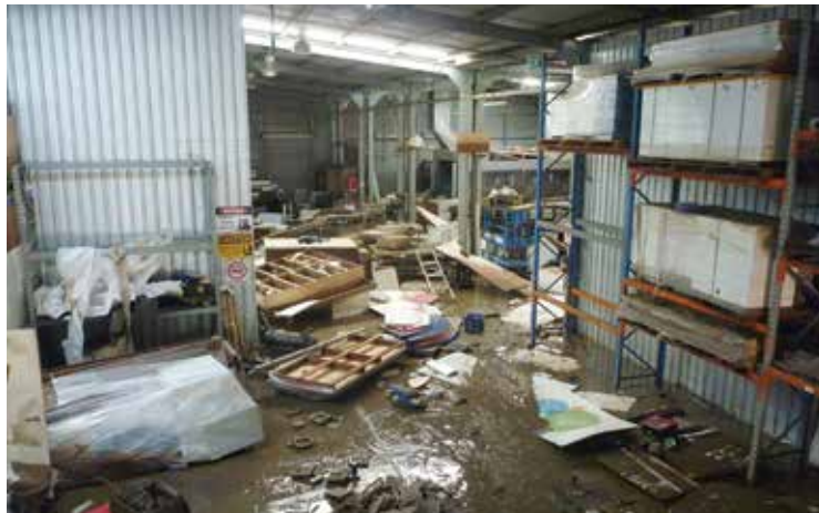
After the waters receded, the inside of the iCatchers building
