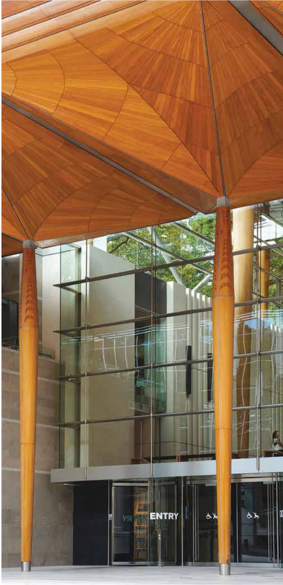
Fifteen metre kauri encased columns support the impressive kauri canopy.
