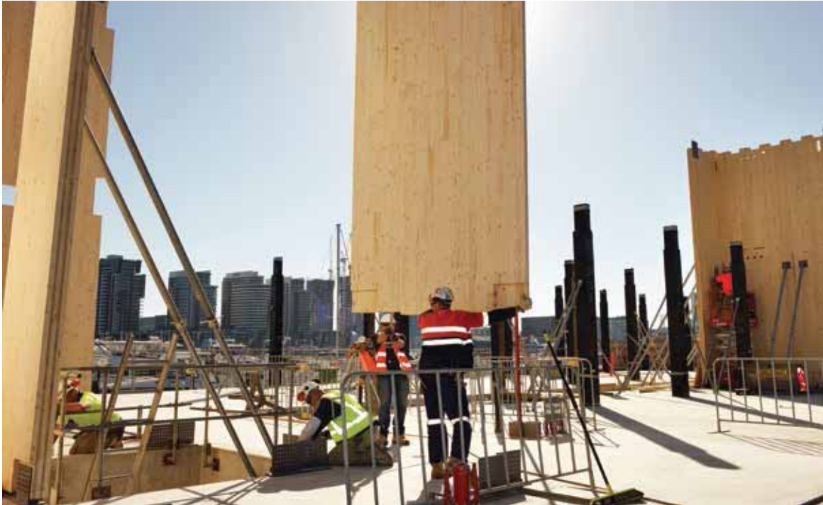
Positioning CLT panels
