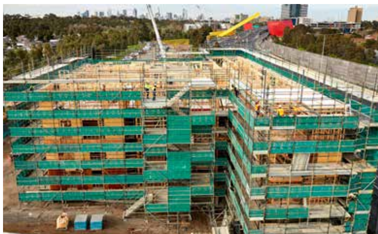
The Green under construction in Melbourne. Mid-rise buildings using lightweight and massive timber construction systems provide opportunities for all types of timber products.
