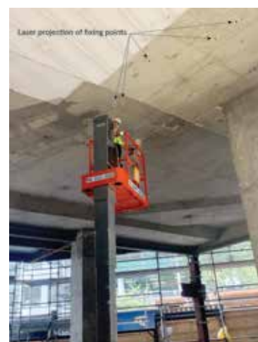
The Flexijet 3D laser beam shows the fixing points on the ceiling with millimetre precision. Just follow the laser and mark the spot.
